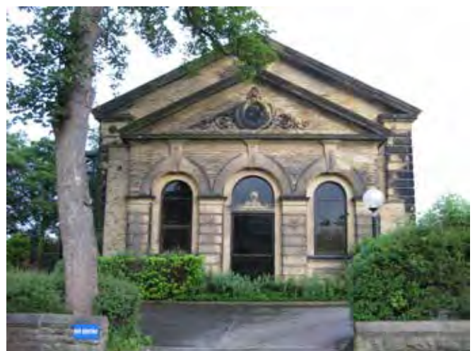
Fig. 2.10 Former Methodist chapel in Shadwell La
