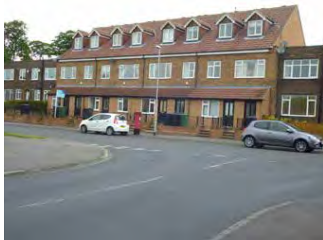
Fig. 3.59 Shops converted to residences in High Moor Cres
