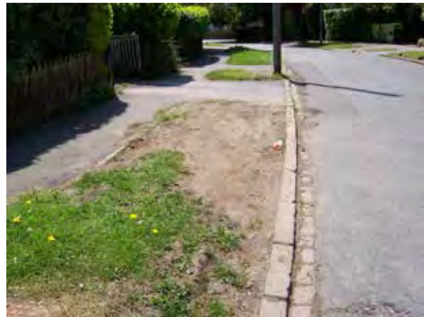
Fig. 3.25 Grass verge damaged by parking
