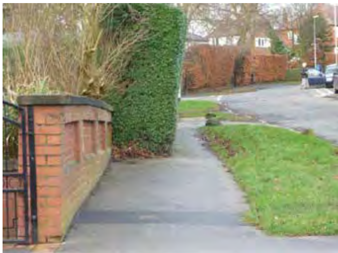
Fig. 5.12 Hedge overhanging footpath
