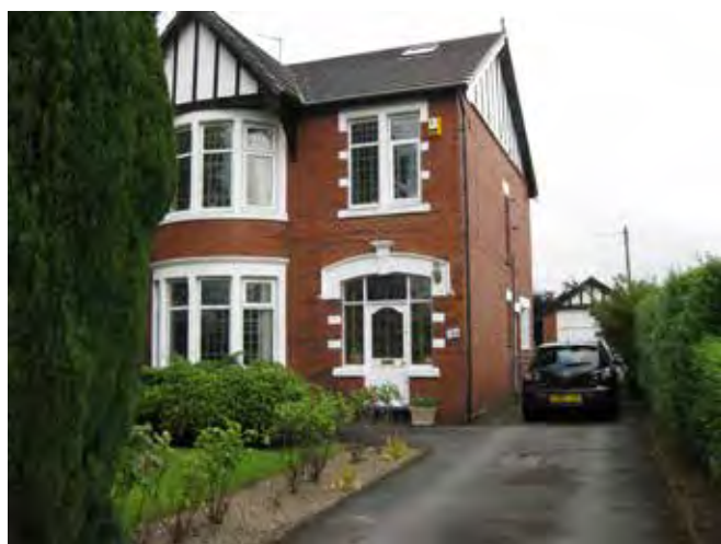
Fig. 3.49 Semi-detached house in Street Lane
