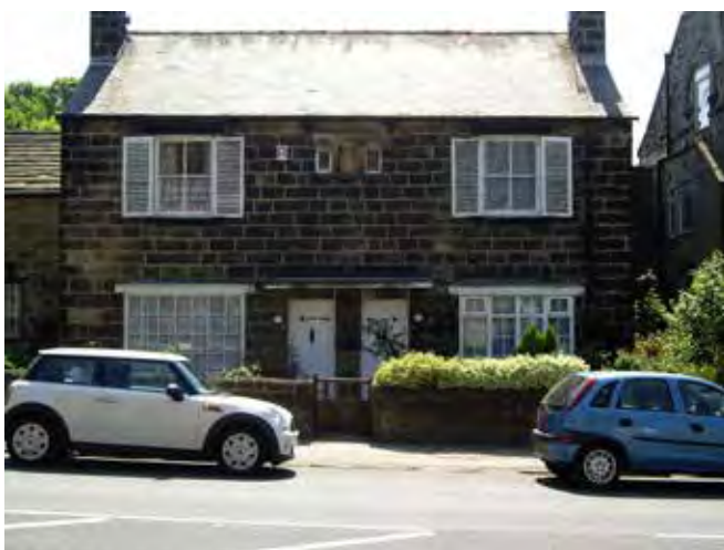
Fig. 3.81 Stone cottages at nos 284, 286 Harrogate Rd
