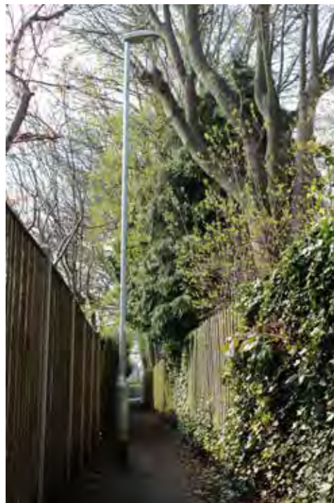
Fig. 5.13 Lamppost obstructing footpath (now repositioned)
