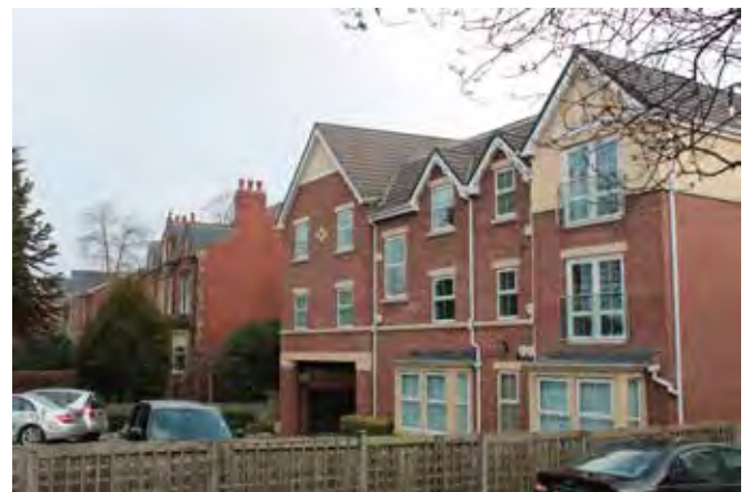
Fig. 3.5 Match of style of new apartment building to Victorian villas in Harrogate Rd
