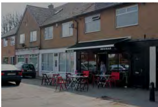
Fig. 6.6 Retail units at Chelwood Drive
