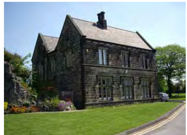
Fig. 3.80 Roman Catholic presbytery adding greatly to the pleasant character of the area.
