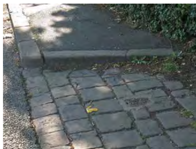
Fig. 5.11 Step between footpath and driveway
