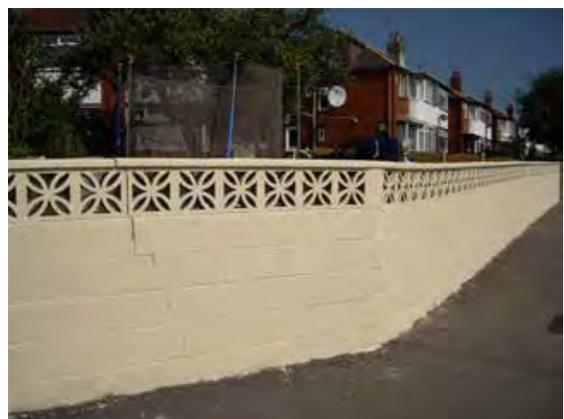
Fig. 3.27 Boundary wall not in keeping with surroundings
