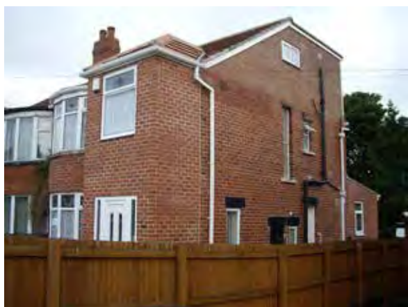
Fig. 3.20 Extension markedly changing original roof line
