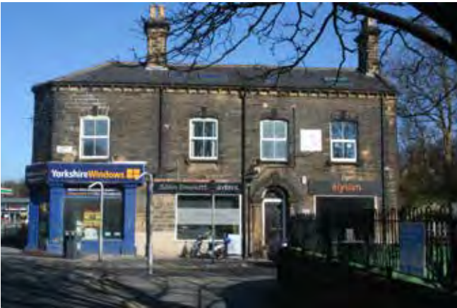
Fig. 3.39 Stone houses on corner of Sand Hill La
