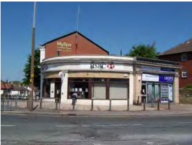
Fig. 3.32 Art deco style HSBC building
