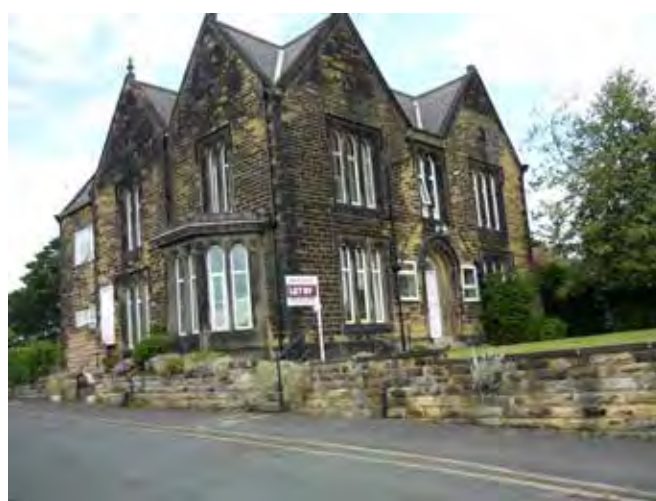
Fig. 3.84 Victorian villa in Allerton Grange Walk
