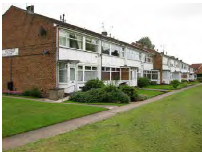
Fig. 3.60 High Moor Court to residential accommodation may be suitable here in future and the parade would benefit from landscaping.
