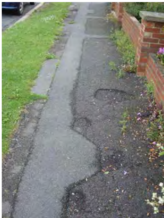
Fig. 5.7 Irregular footpath due to degradation
