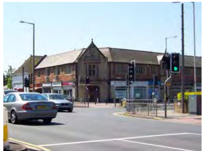
Fig. 6.4 The Corner House (former casino) and retail outlets below at Moortown Corner
