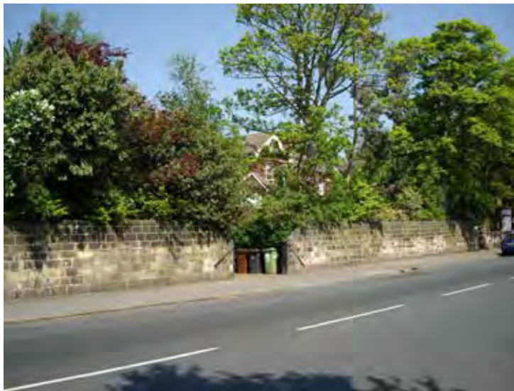
Fig. 3.18 Original stone wall in Harrogate Road
