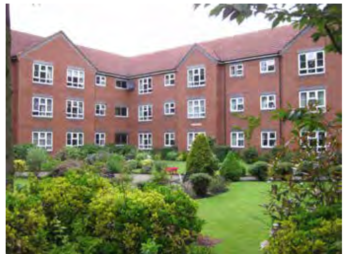
Fig. 3.55 The Spinney - apartment building
